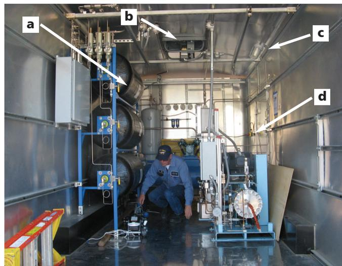
**Photo 6:** Missouri S&T's mobile hydrogen unit showing a) compressed hydrogen tanks; b) ventilation system; c) warning light; and d) emergency shutoff button. Not visible in this picture are hydrogen sensors and another emergency shutoff device located on the outside of the trailer.
