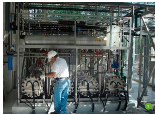
1 1.5 MW PEM cell stack developed by Hydrogenics
